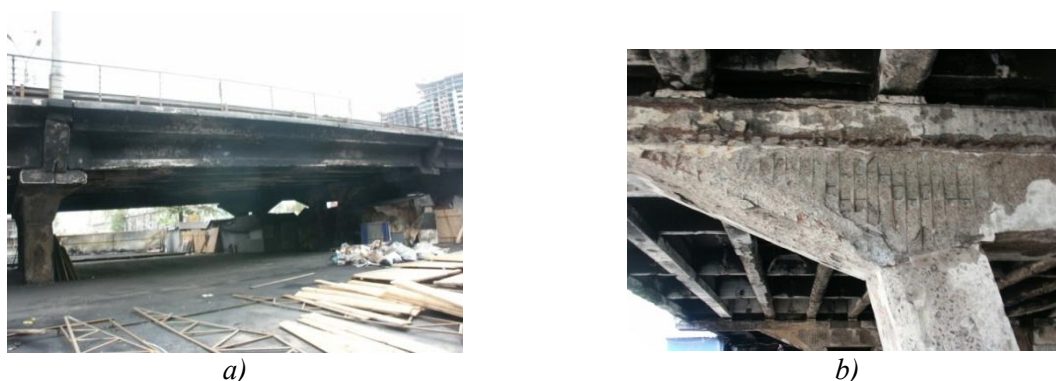
Figure 1 – Overpass structures near the Shulyavskaya metro station in Kyiv after a fire
